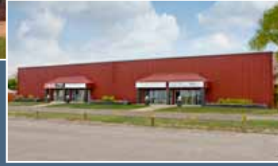
The Hargreaves Building
